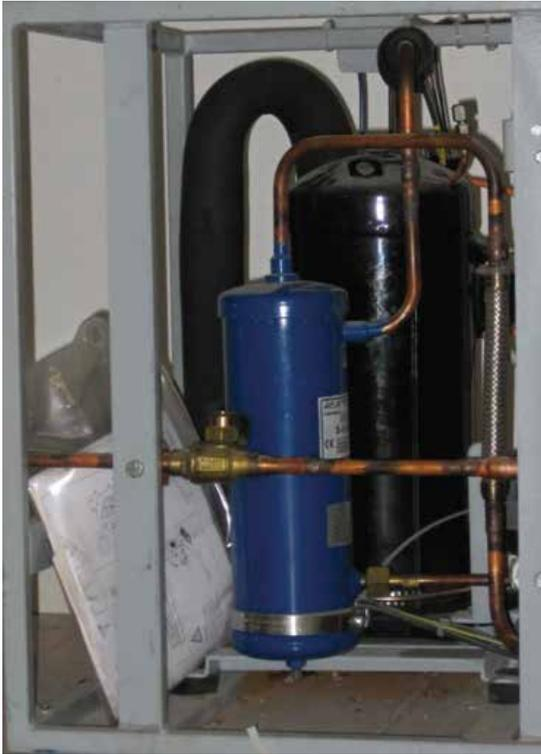
Fig. 4: Copeland scroll compressor for deep freezing
