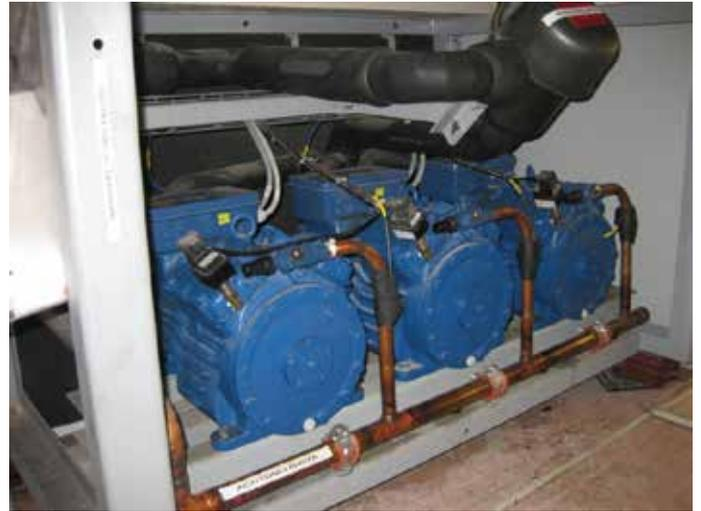
Fig. 2: Compound system with 3 Bock compressors
